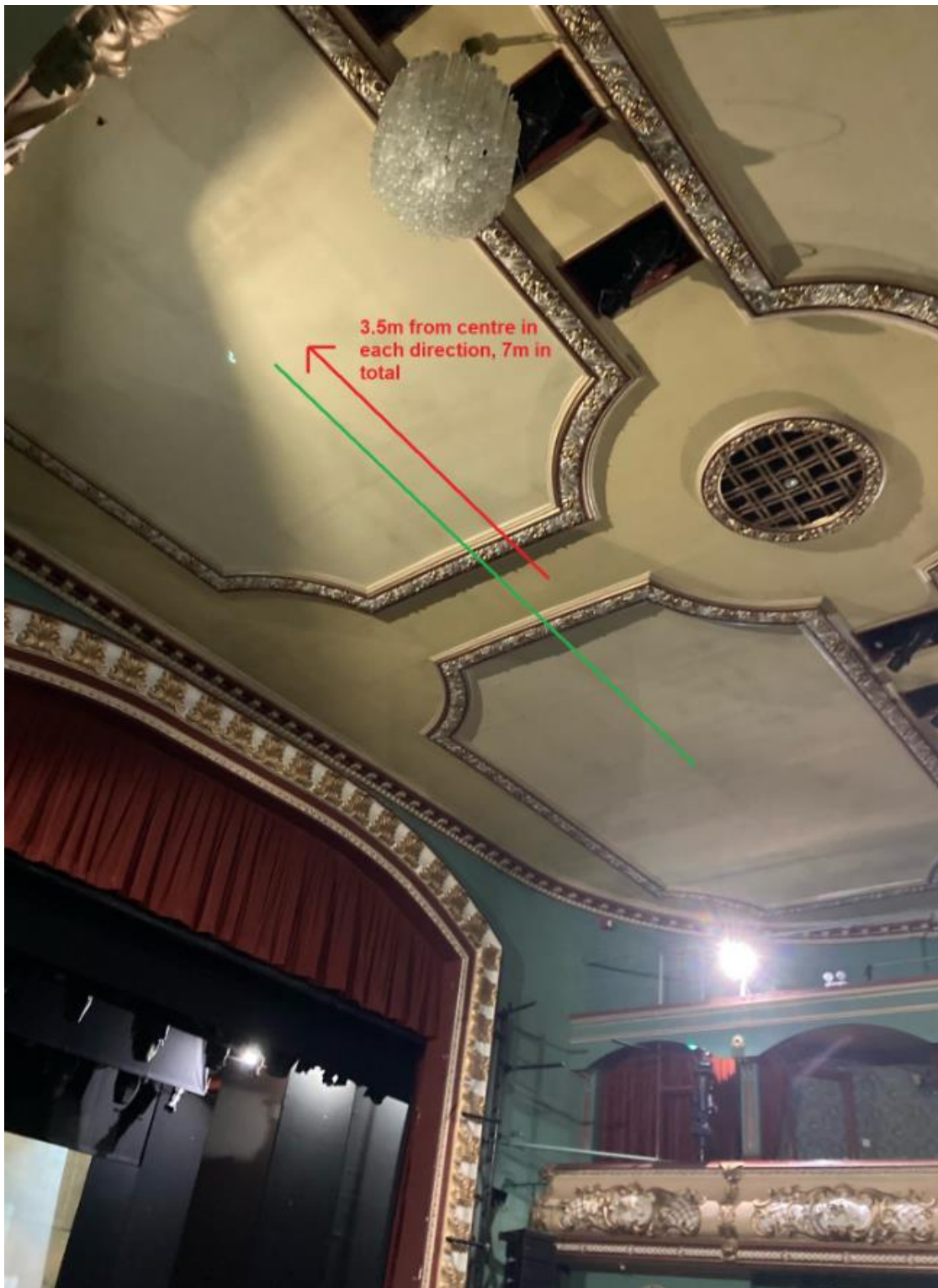
Photograph showing where the lighting rig will be installed.
